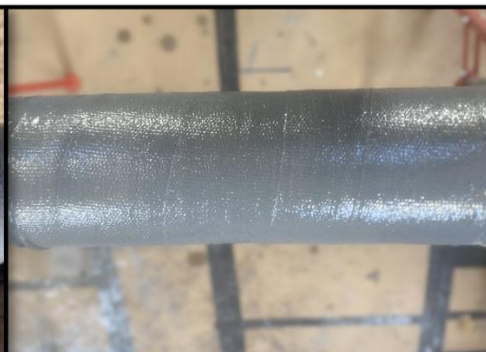
Allow to cure a minimum 2 hrs.
