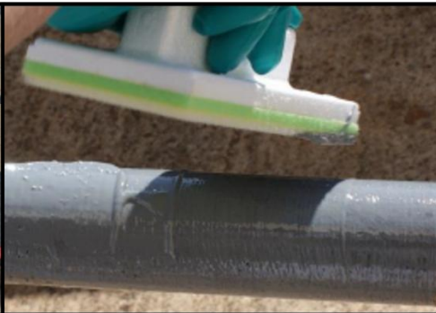
Apply epoxy 10-15 mils thick
