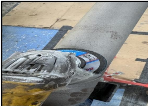
Surface prep pipe to white metal
