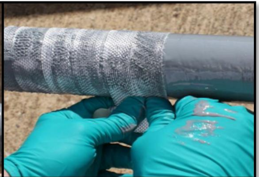
Overwrap fabric with 50% overlap
