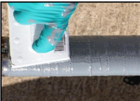
Apply a second layer of epoxy
