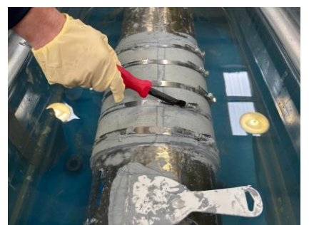
Tighten System and Cure
