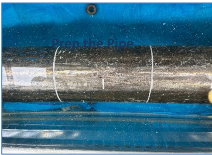
Prep the Pipe
