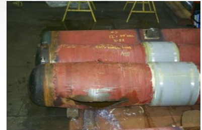
Pipe Body Failure @ 4,260 psi
